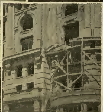
Effect of Fire on Exterior Materials
